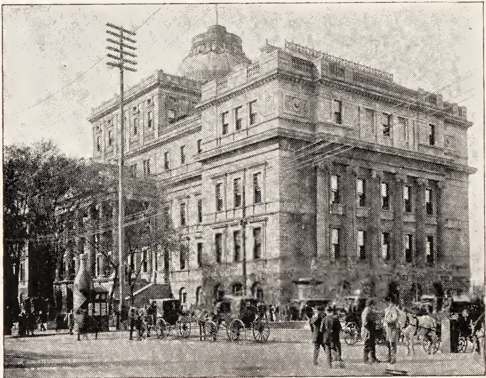
COURT HOUSE, MONTREAL.
